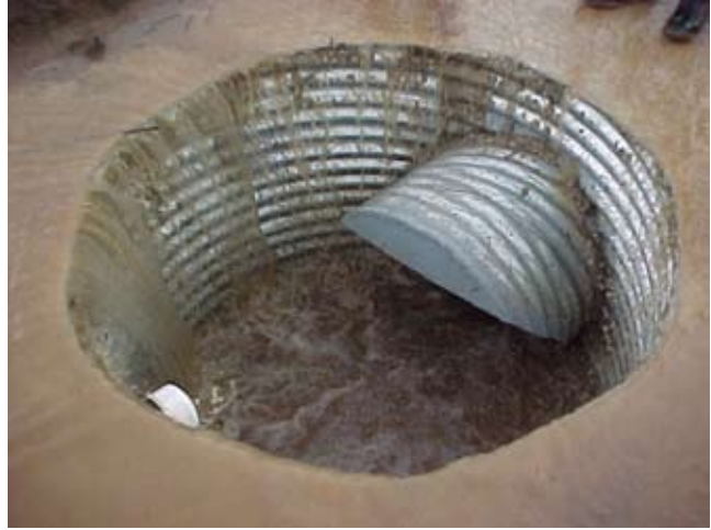
Figure 13–37 Riser with canopy barrel inlet
