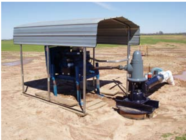
Figure 13–20 Hydrology enhancement with pumped ground water
