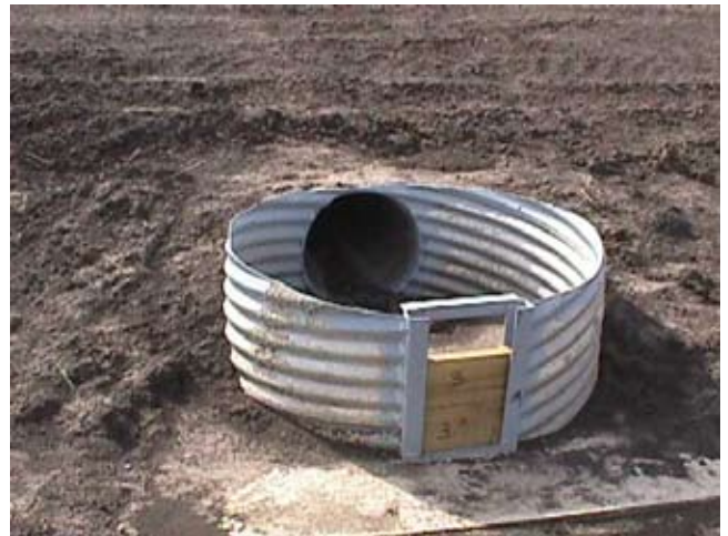
Figure 13–35 CMP riser with stoplogs
