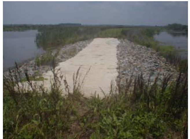
Figure 13-39 Armoring auxiliary spillway with concrete and riprap
