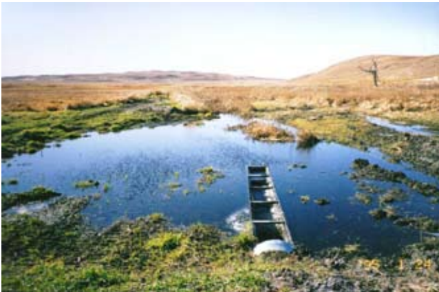
Figure 13–30 Cut pipe culvert
